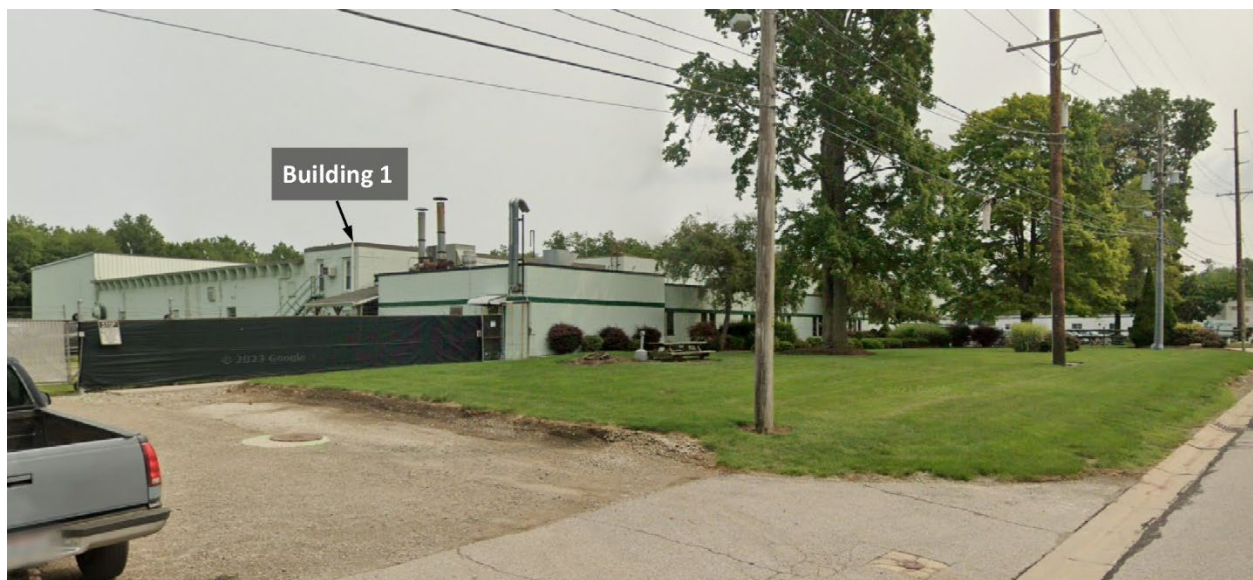
Figure 3. Approach from the West on Schneider Court-Building 1 Alpha/Bravo Corner
