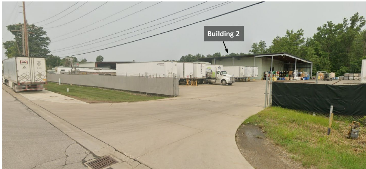
Figure 6. Building 2 Alpha/Delta Corner
