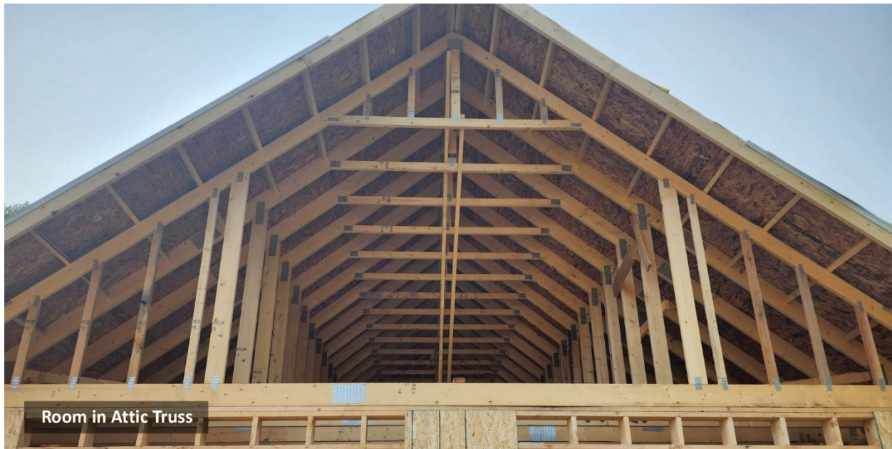
Figure 13. Room in Attic Truss
